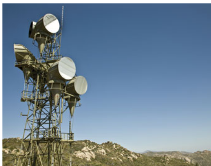
FIGURE 8.17 Any information that can travel over a telephone or coaxial cable can be transmitted via microwave.
